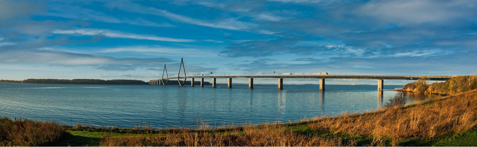
The Farø Bridges are two road bridges that connect the islands of Falster and Zealand in Denmark by way of the small island of Farø Photo: iStock
