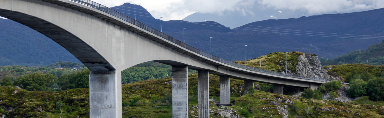
Herøy bridge connecting Gurskøya and Leinøya, Norway
