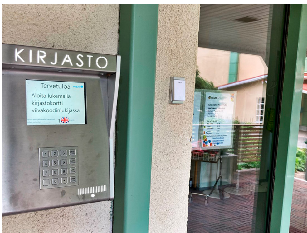
Kinnula's library and the entrance code system used outside of opening hours.
